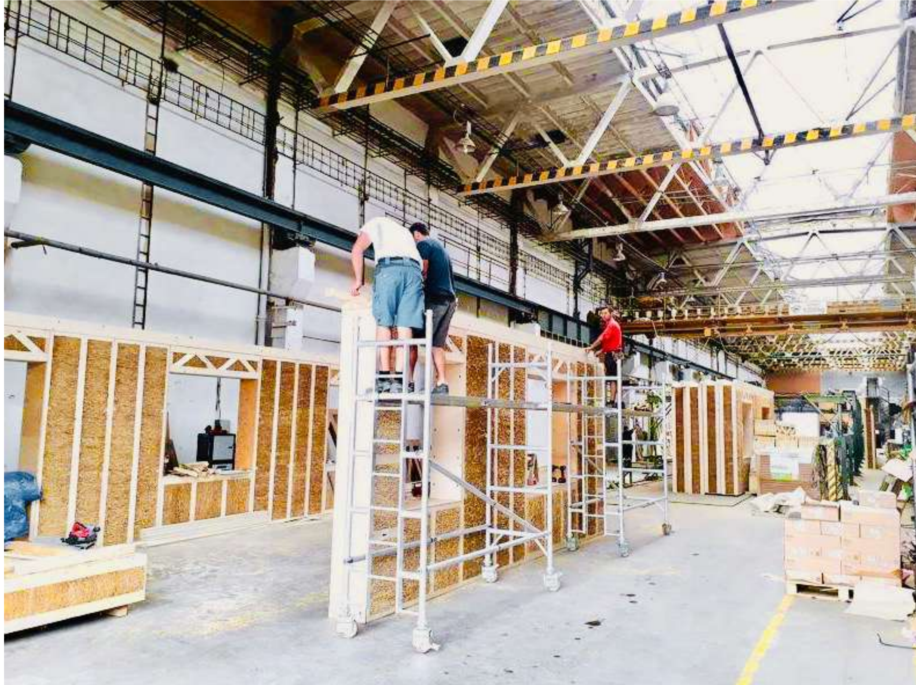
Pre-assembly in a hall
